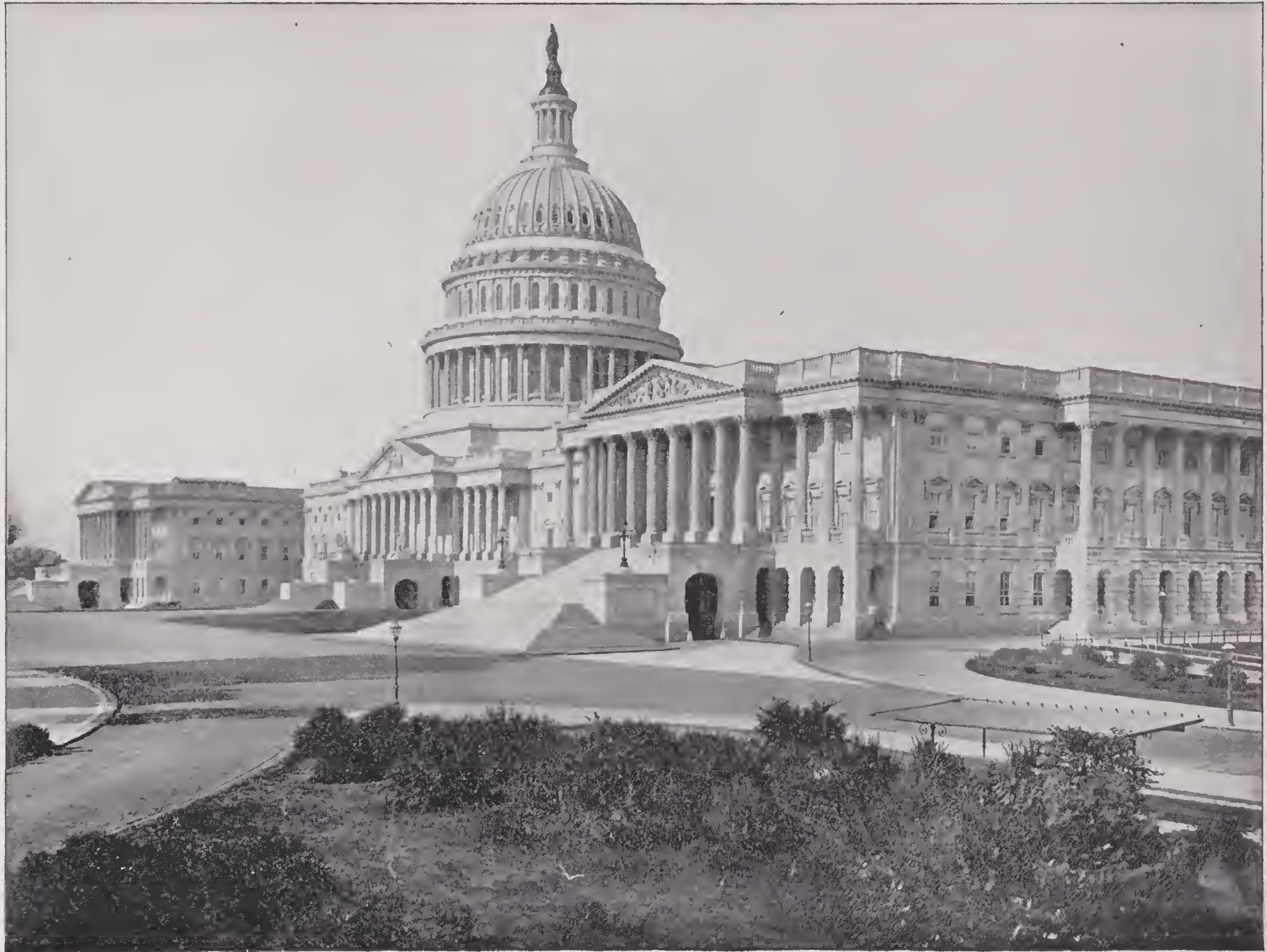
THE CAPITOL, WASHINGTON, D. C.—The Capitol in Washington deserves a foremost place among the first buildings of the world. It stands upon an eminence in the midst of extensive grounds. The general plan is that of a central building, surmounted by a dome, flanked by two wings. The length of the structure is seven hundred and fifty-one feet, the breadth ranging from one hundred and twenty-one to three hundred and twenty-four feet at the different parts, the whole covering three and a half acres. Its extreme height from the ground to the top of the Statue of Liberty, which stands upon the dome, is three hundred and seven and a half feet. The entire cost of the building has been $13,000,000.
